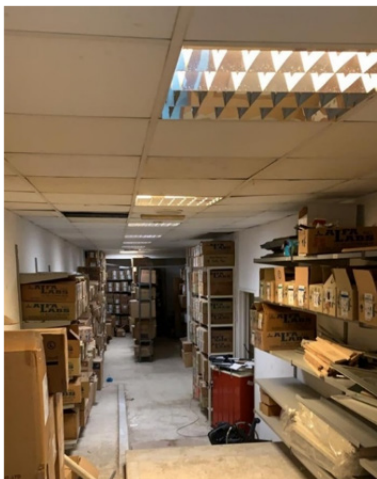
Figure 27 - Lighting system condition in Tripoli Public Hospital
